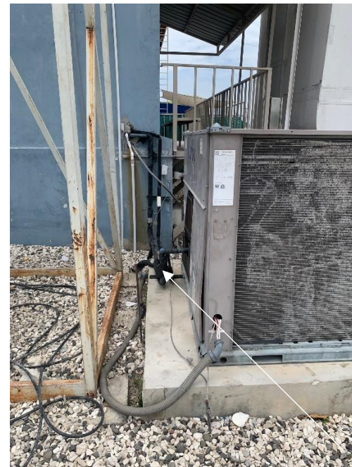
Outdoor unit connection to Indoor unit
