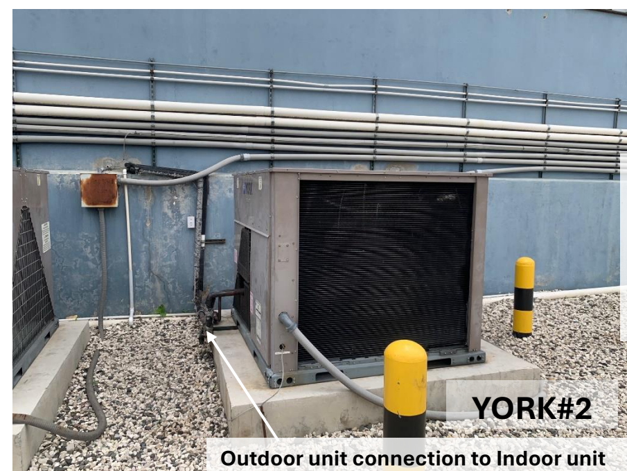
Outdoor unit connection to Indoor unit
