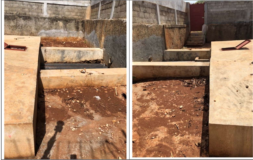
Figure 4. Sediment at base of capture structure east side (left) and west side (right)
